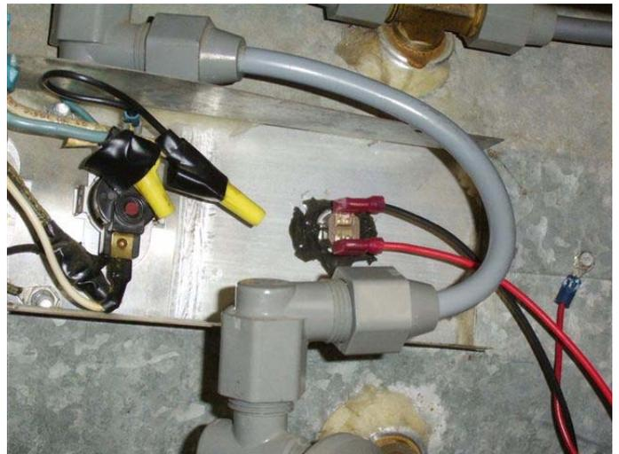
This kit is designed to close the engine hot water loop when the water in the hot water heater reaches 140 degrees.
