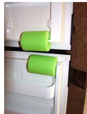
Section of a swim floatie to keep refrigerator open when not in use to help prevent mold.
