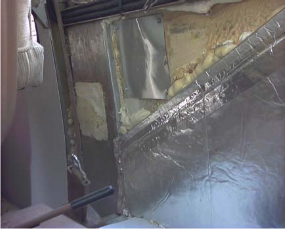
The flashing is secured with pop-rivets at the corners within the recesses of the panel.
