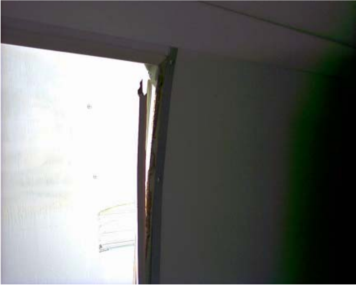
The original door molding had turned yellow, brittle and had fractured in several places.
